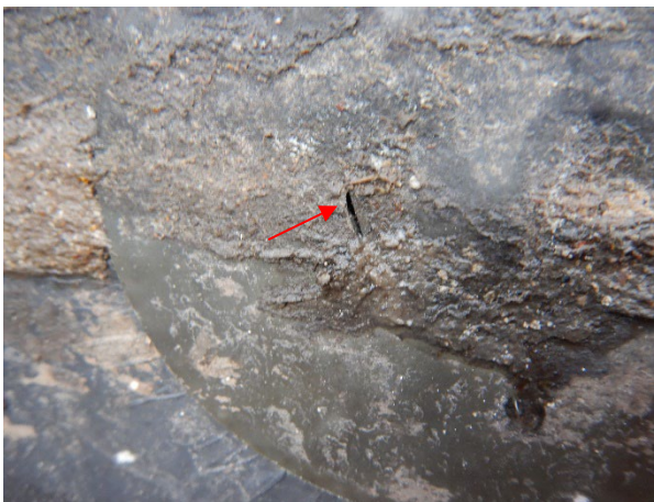
Foto 3.49: Beschadiging in afdekking bevestigingsring.
