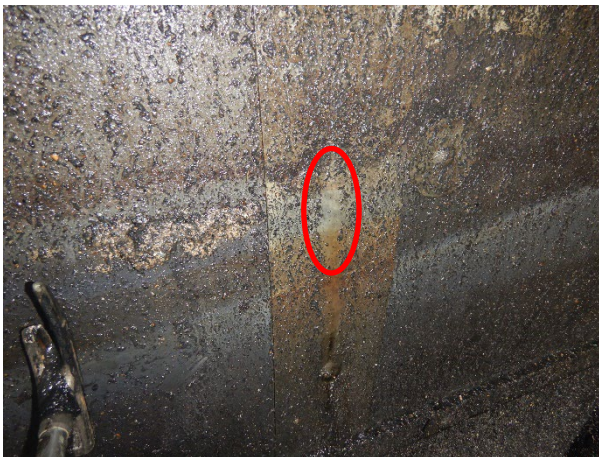
Foto 3.34: Scheurtje in HDPE-lining.
